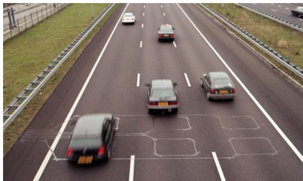
Figure 3.1: An example image of loops in the road, from www.heijmans.nl/ . These loops are used to measure the speed and intensity of traffic driving over it.
