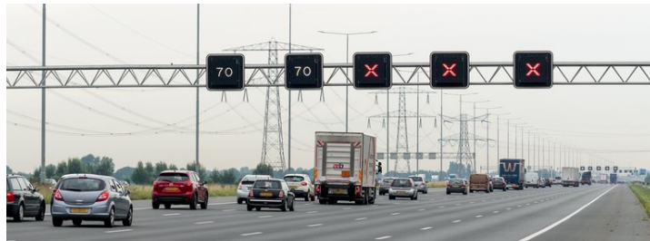
Figure 3.4: An example of a road situation, shown by matrix signs, from www.autoblog.nl/ . In this situation, there are two open lanes with a maximum allowed speed of 70 km/h. In my model, this would reflect as [70, 70, 0, 0, 0, 0] .
